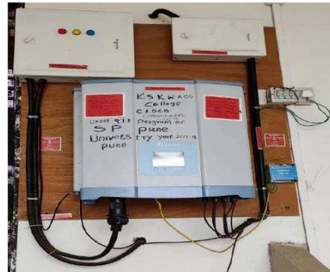
Solar on Grid Inverter (15.3KW)
