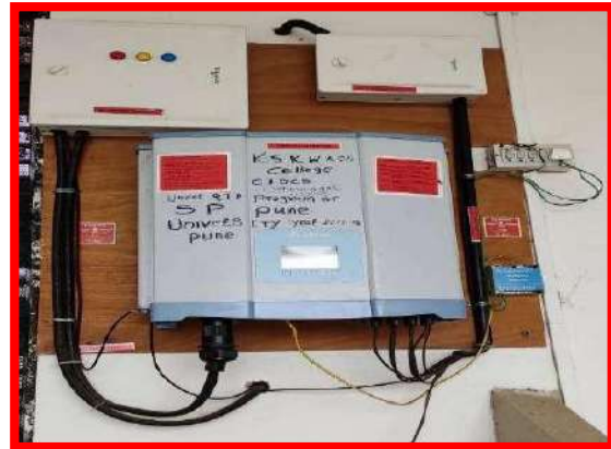
Solar - On Grid Inverter System (15.3KW)
