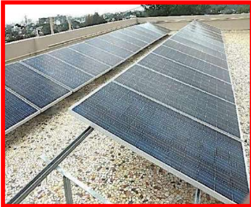
Solar - On Grid Inverter System (15.3KW)
